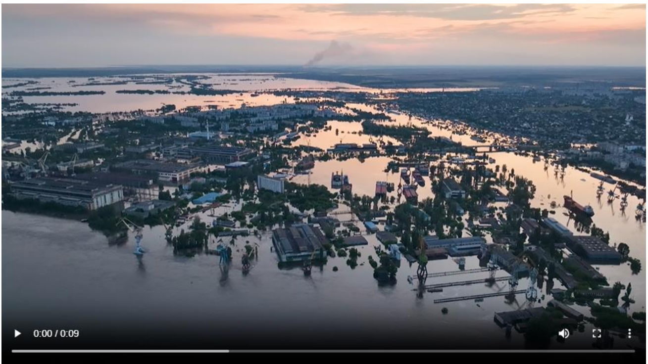
Fig. 5. The city of Kherson after the explosion on the Kakhovka Dam. © Vladimir Smirnov on Adobe Stock. All rights reserved.
